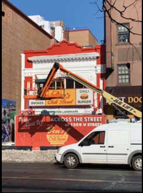
Ben's Chili Bowl Original U Street NW Location Currently Under Construction
