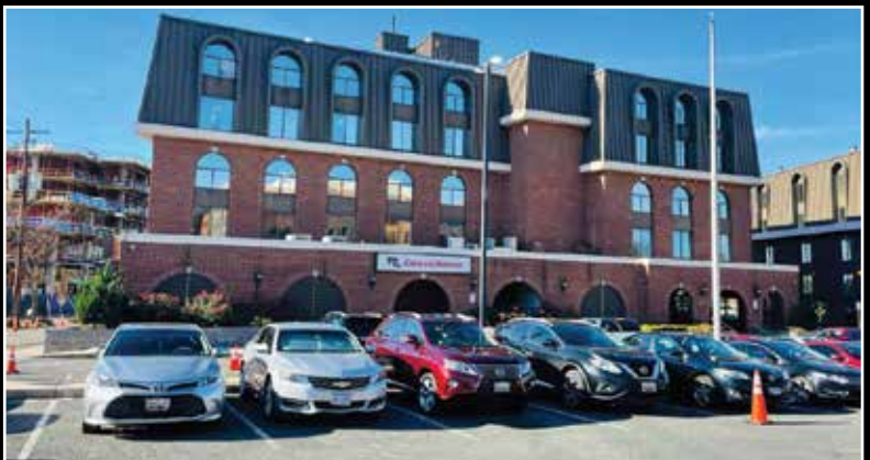
This is the Court Services and Offender Supervision Agency (CSOSA) location on MLK Avenue. Readers who will be on supervised release after returning home to SE Washington, DC, will likely report here. Notice the construction you can see to the left—a reminder of the aforementioned gentrification of Anacostia!
